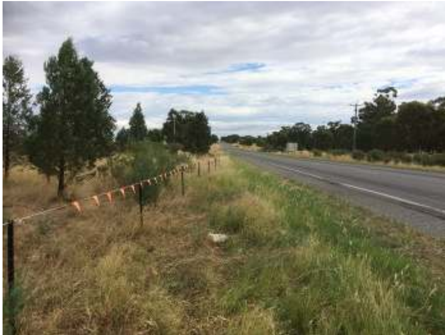
Figure 7-3 Example of exclusion zone fencing.
