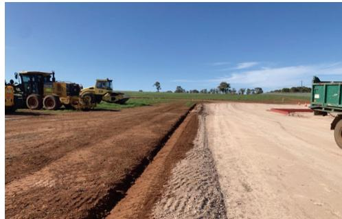
**Photo 32:** Site access area: Upslope 'clean water' diversion drain without adequate erosion and sediment control measures.
