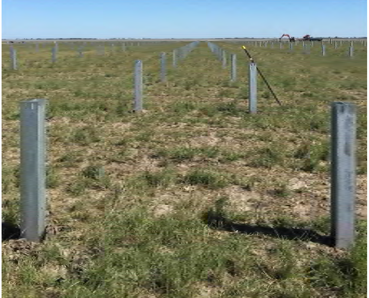
Figure 4-2 Piling installation for a single axis tracker
