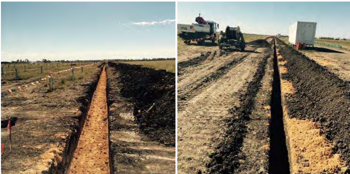
Figure 4-8 Examples of underground cable trenches with bedding sand installed.
