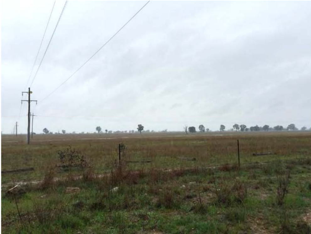
Figure 4-7 Example TransGrid transmission line.
