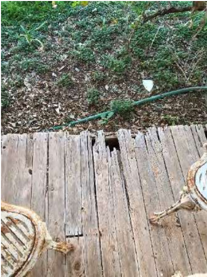
Plate 131. Deteriorated section of the timber verandah decking.
