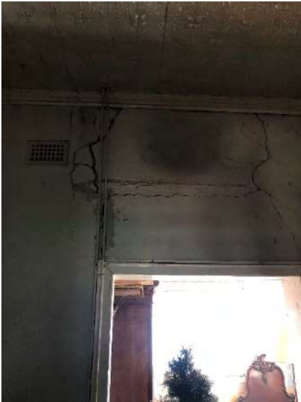
Plate 67. Substantial cracking over the door arch leading to bedroom 4.
