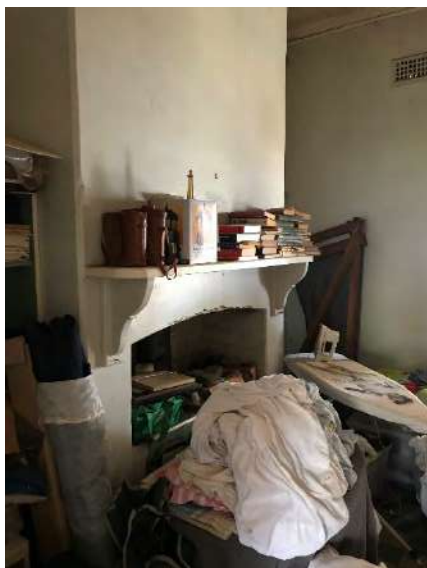
Plate 63. Original kitchen fireplace. This fireplace backs onto the fireplace in bedroom 3 and shares the same flue.
