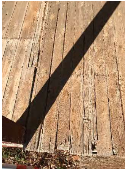
Plate 116. Deteriorated section of some of the hardwood decking on the verandah surrounding the house.
