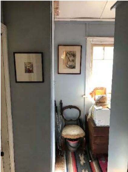
Plate 55. Fibro walls of the ante-chamber room. This area would have been originally part of the wrap around verandah of the house. The area was subsequently enclosed to provide additional floorspace internally.
