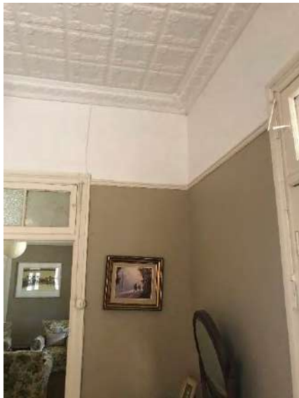
Plate 35. Picture rail and pressed tin ceilings. Pressed metal ceilings are an element of the Federation style of building.
