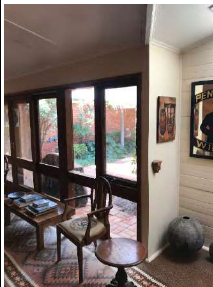
Plate 78. Verandah was originally enclosed in fibro sheeting. The current owners removed the fibro and replaced it with floor to ceiling windows.
