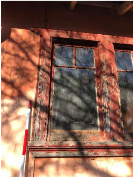
Plate 155. Deteriorated windows within the enclosed verandah section of the homestead.
