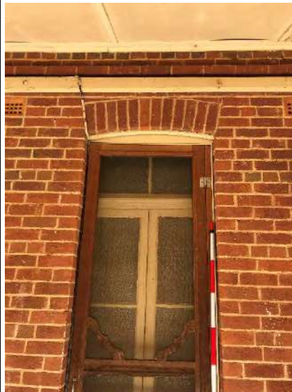
Plate 118. External original window along western façade of the house. Decorative brick arch above the window.
