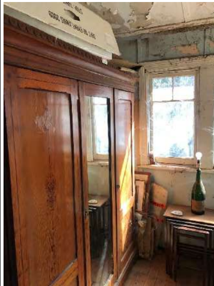
Plate 70. Peeling ceiling and wall paint in bedroom 4 off the original kitchen.
