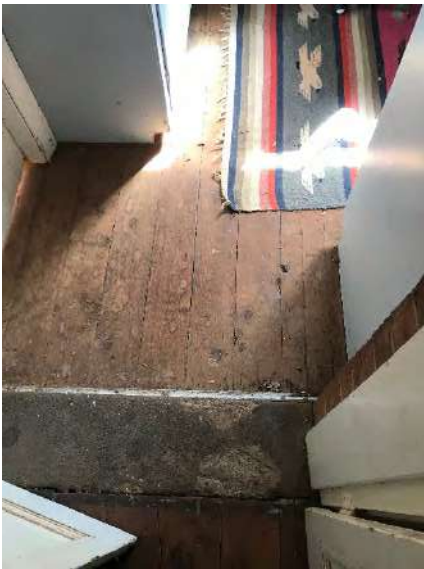
Plate 53. Polished wooden floors of bedroom led into rough floorboards in the ante-chamber, formerly part of the verandah.
