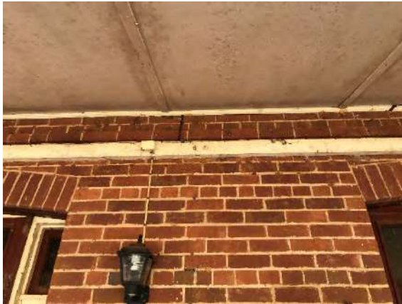
Plate 123. Current electrical wiring along the southern (front) façade of the homestead.
