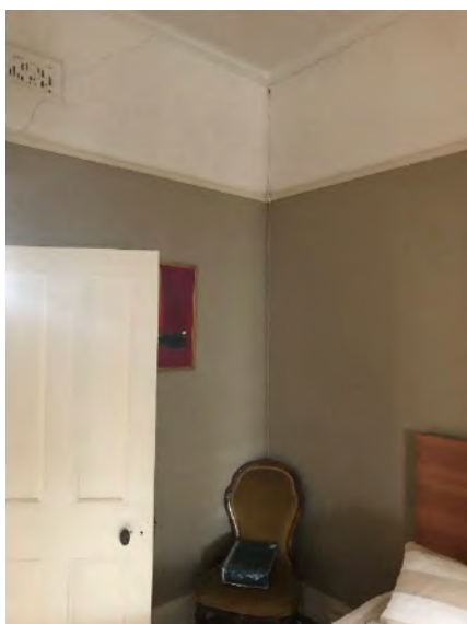
Plate 49. Minor cracking near the wall vent.
