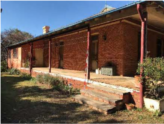
Plate 115. Western side of the house with part of the verandah enclosed to create more internal floor space. Note the absence of decorative woodwork. The posts supporting the verandah are square and do not contain any specific wood patterns. In contrast Nanima homestead has some carving work on its verandah posts and some decorative wood patterns on the protruding gable at the front.
