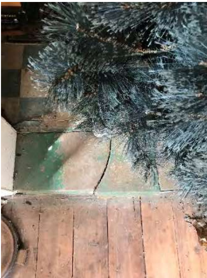
Plate 69. Cracked concrete step leading from lino-lined kitchen onto the rough hardwood floor of bedroom 4.
