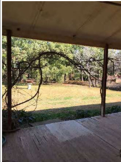
Plate 130. Section of the deck along the southern (front) façade that has required replacement due to deterioration. Lack of decorative elements along the verandah.
