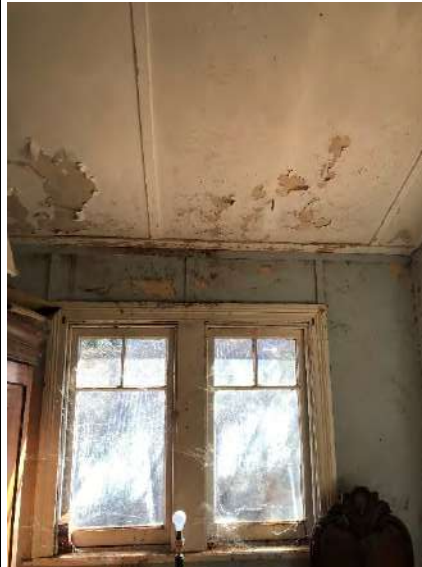
Plate 72. Peeling ceiling paint.
