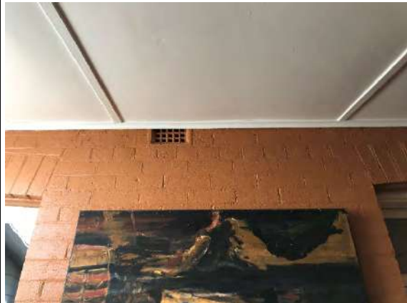
Plate 76. Original external wall vent partially covered by the new fibro ceiling installed in the gallery.
