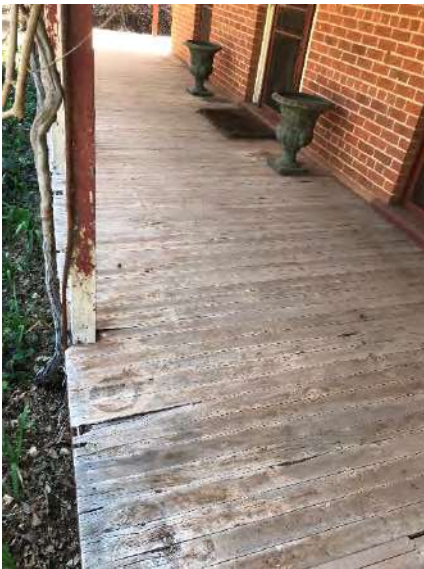
Plate 129. Decking along the southern verandah has deteriorated and begun splintering apart
