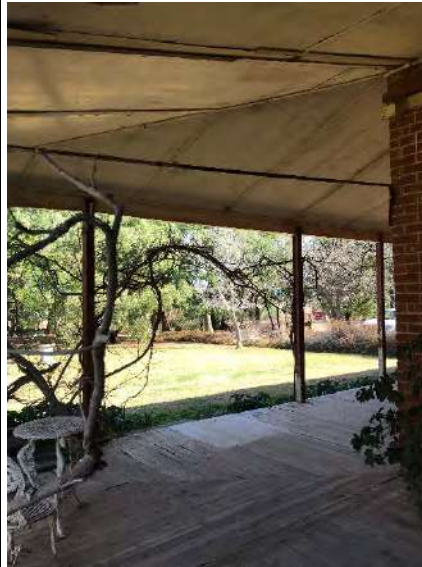
Plate 132. Fibro roof sheeting along the verandah requires replacement due to deterioration.
