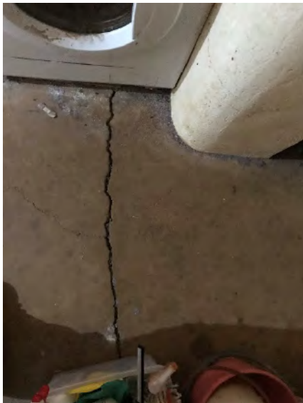
Plate 97. Cracked concrete floor.
