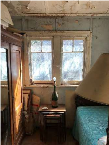
Plate 71. Windows that were installed with the enclosure of the balcony.
