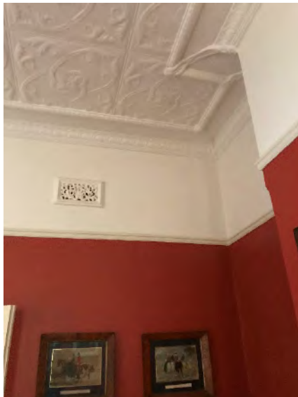
Plate 13. Picture rail and pressed tin ceilings. Pressed metal ceilings are an element of the Federation style of building.
