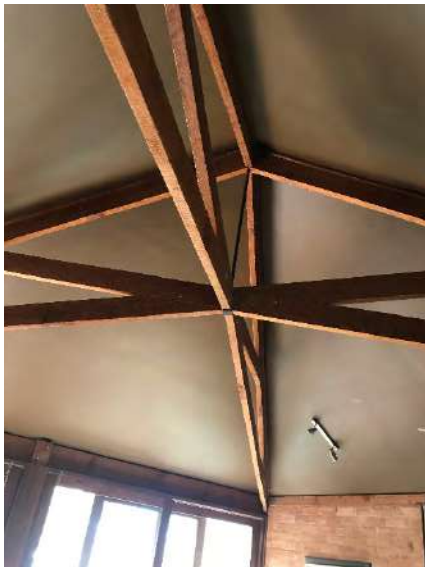
Plate 7. High vaulted ceiling with scissor truss.
