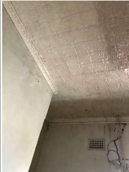
Plate 68. Pressed tin ceilings. Pressed metal ceilings are an element of the Federation style of building.
