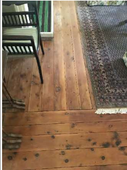
Plate 28. Floorboards internally within the room placed perpendicular to the others. Originally the room would have included an internal wall for a hallway.
