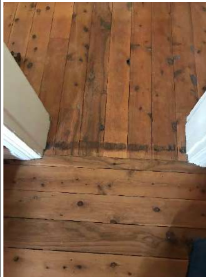
Plate 18. Flooring from dining room into the living room. Note the change in direction of the floor boards.
