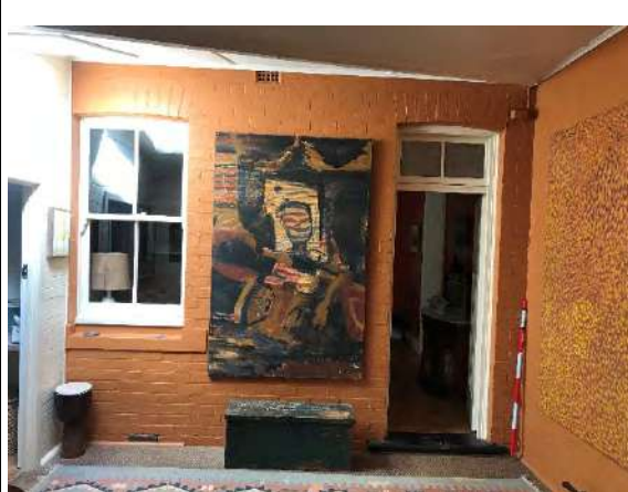
Plate 75. Original external brick wall of the homestead with external door and window. The original wrap-around balcony has subsequently been enclosed and used for an art gallery.
