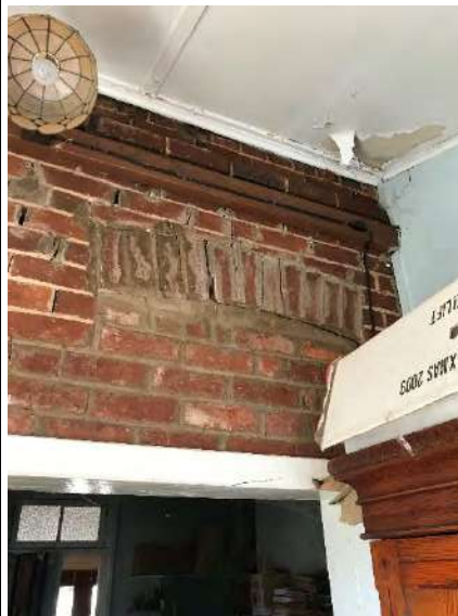
Plate 74. Original external doorway to the verandah removed and replaced with a wider doorframe.
