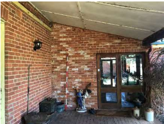
Plate 133. Kitchen extension on the eastern façade of the building. The sandstock bricks used in the extension were sourced from a property on Dubbo.
