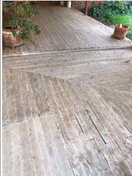
Plate 128. Decking along the southern verandah. Some areas of deterioration and splintering.
