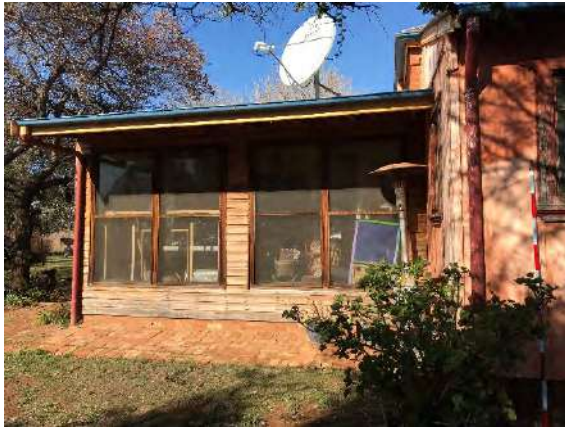
Plate 153. Western façade of the weatherboard art gallery extension. Note the change in the roofline. Art studio is situated just to the north of the enclosed verandah area.
