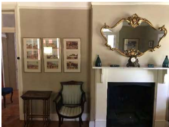
Plate 23. Original fireplace refurbished. This fireplace backs onto the one in the dining room and shares the same flue.
