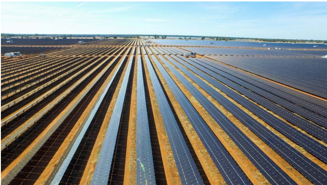
Figure 4-1 Typical fixed array solar plant - Nyngan NSW (Nyngan Solar Plant is owned by the Powering Australian Renewables Fund (PARF). Image courtesy of PARF).
