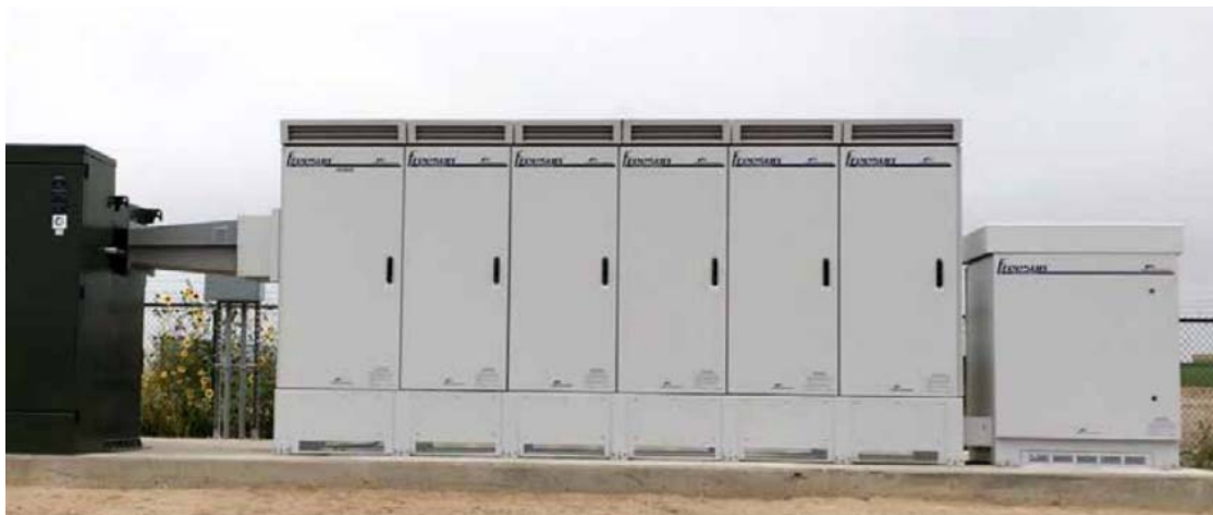
Figure 4-6 Typical PCS (courtesy: Power Electronics).
