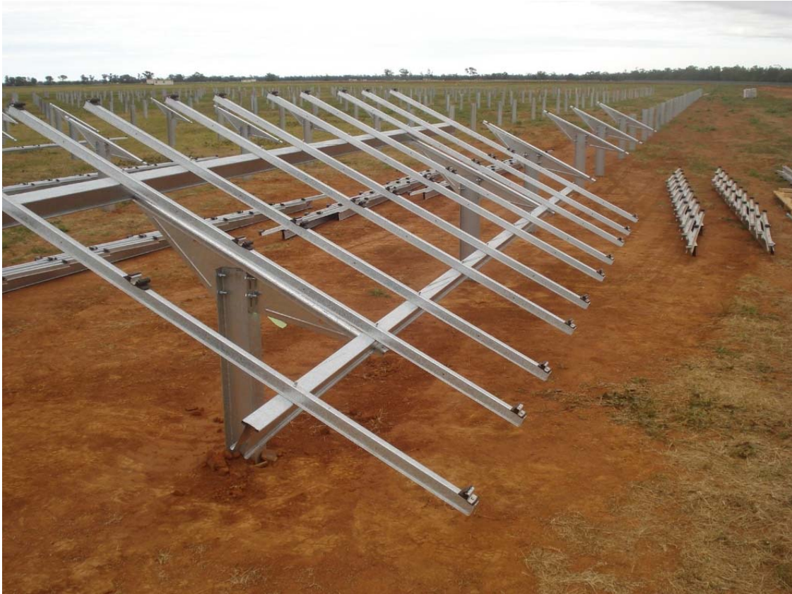
Figure 4-2 Example of typical panel framing (Image courtesy of PARF).
