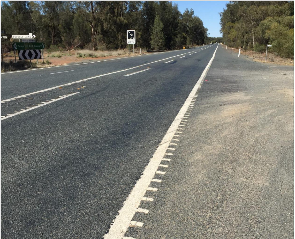
Figure 5: Newell Highway at Bodells Lane (Looking West)
