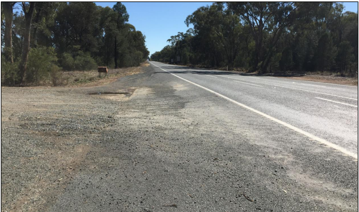
Figure 4: Newell Highway at Bodells Lane (Looking East)
