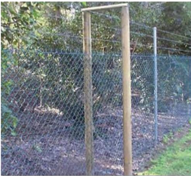
Figure 6.2 An example of the fauna bridge proposed to allow for movement of arboreal fauna over the solar farm security fence
