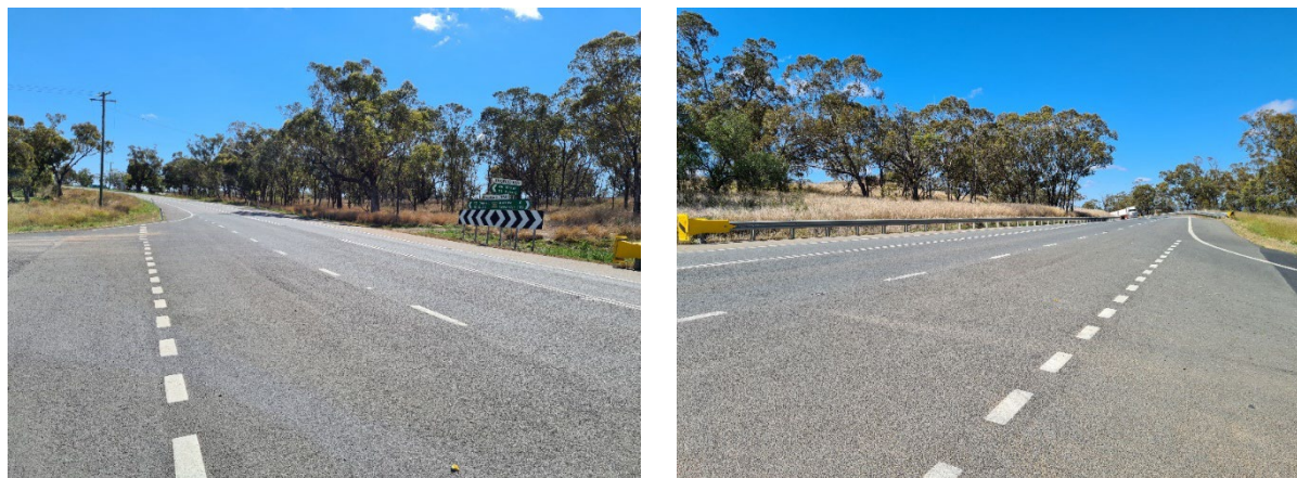
Figure 2-4: Golden Highway looking west (left) and east (right)
