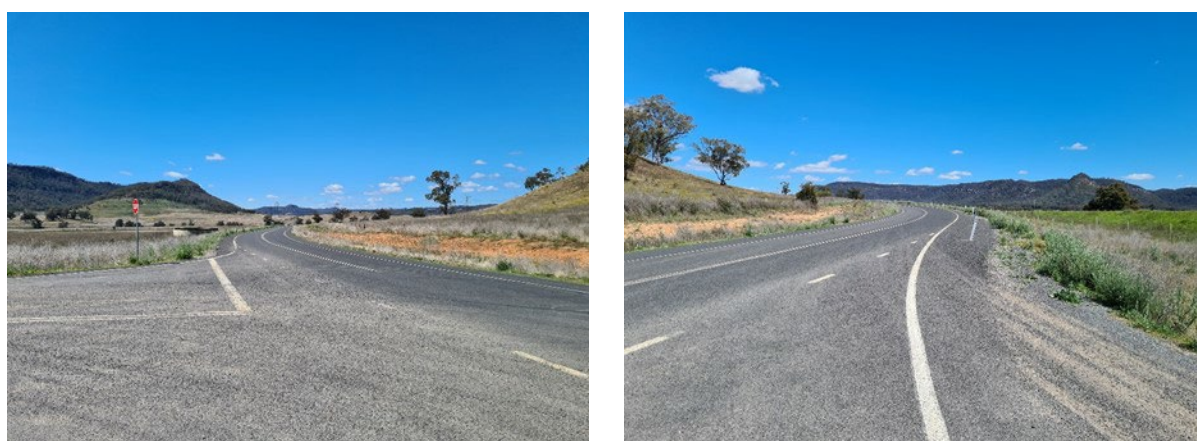
Figure 2-7: Wollar Road looking east (left) and west (right)
