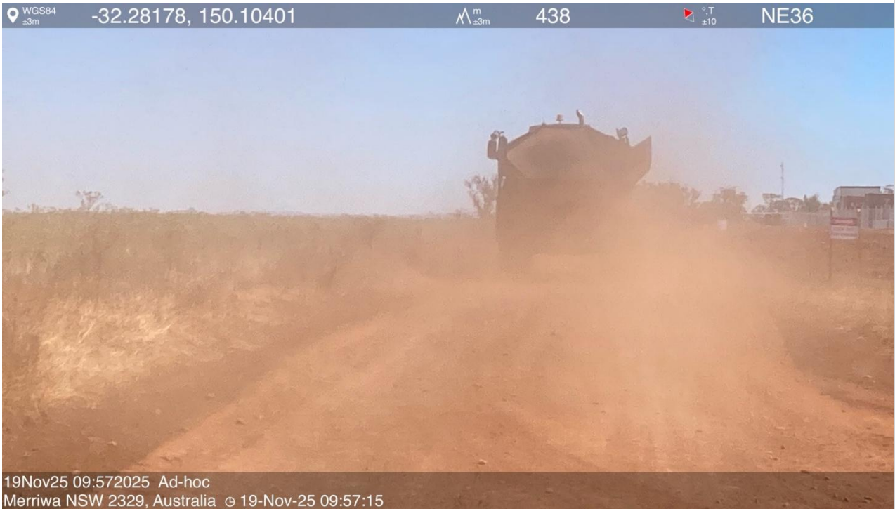
Dust generation from earthworks
