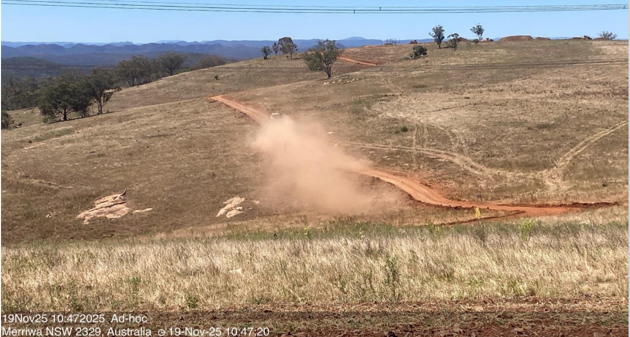
Dust generation from earthworks
