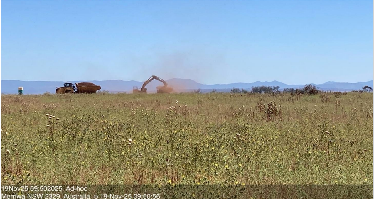
Dust generation from earthworks
