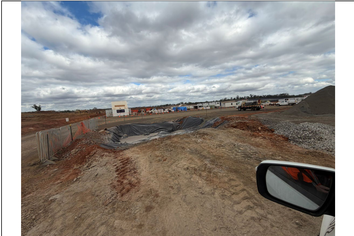
Photo 16 Dedicated concrete washout area at DTI subcontractor compound.
