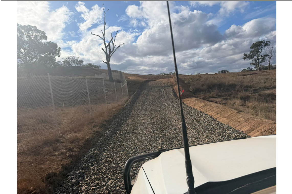
Photo 20 Stage 4, recently stabilised internal acces roads.
