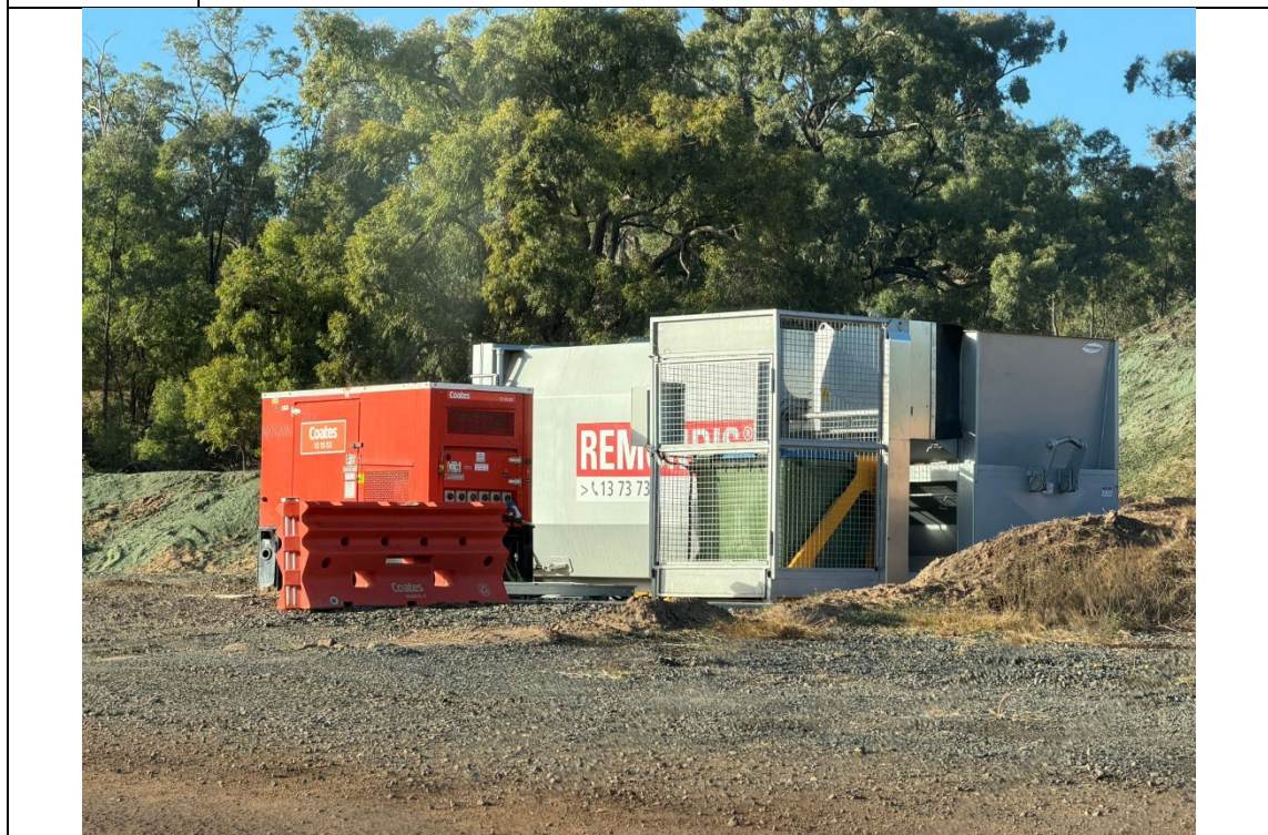
Photo 7 One of several waste compactors on the site to reduce waste volumes and minimise traffic movements.
