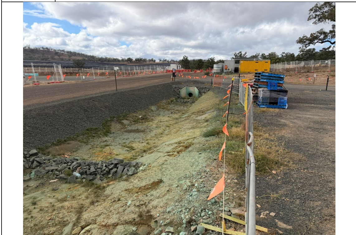
Photo 13 Temporary workers camp, showing polymer applied to swales and rock checks as ERSed controls.
